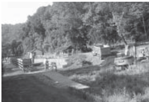
Popple Construction at work at Locks 22-23...
