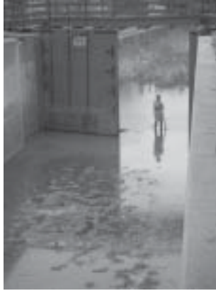
Cleaning up Lock 11—no small task.
