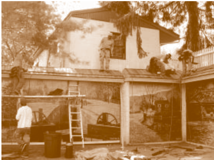
So many workers on such a small roof.
