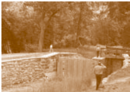
The installation of the stop gate at Rocky Falls created a stir. Photo by Carole Mebus.
